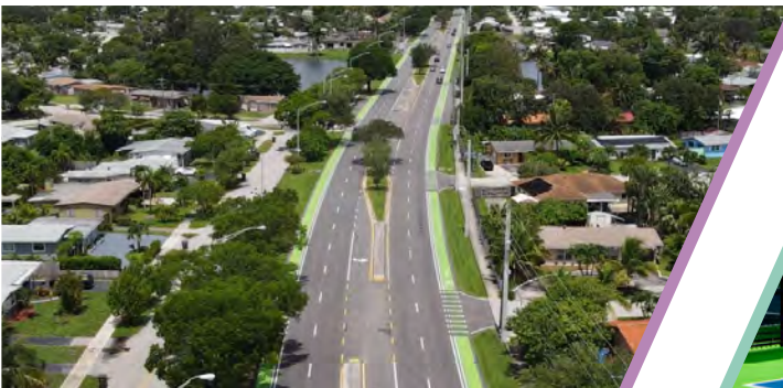
Prospect Road Improvements Enhancement
